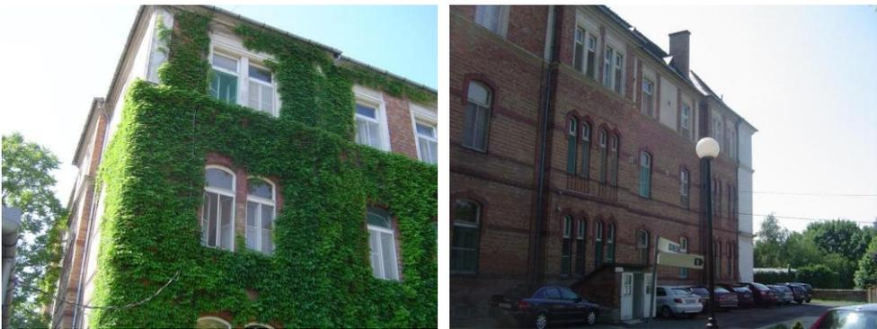
The boundary structure of the building and mechanical engineering structures do not meet current standards. The wooden doors and windows of the building are average 50-year old, the boundary heat transfer factors are higher than the current regulations.
