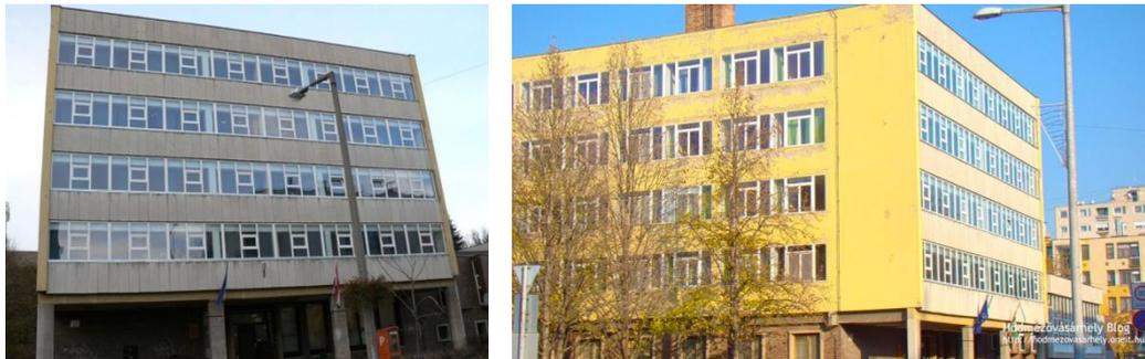
The college was built in 1969. The building is 38 years old, the renovation became necessary, because of the structure of the cooling surface and the windows.
