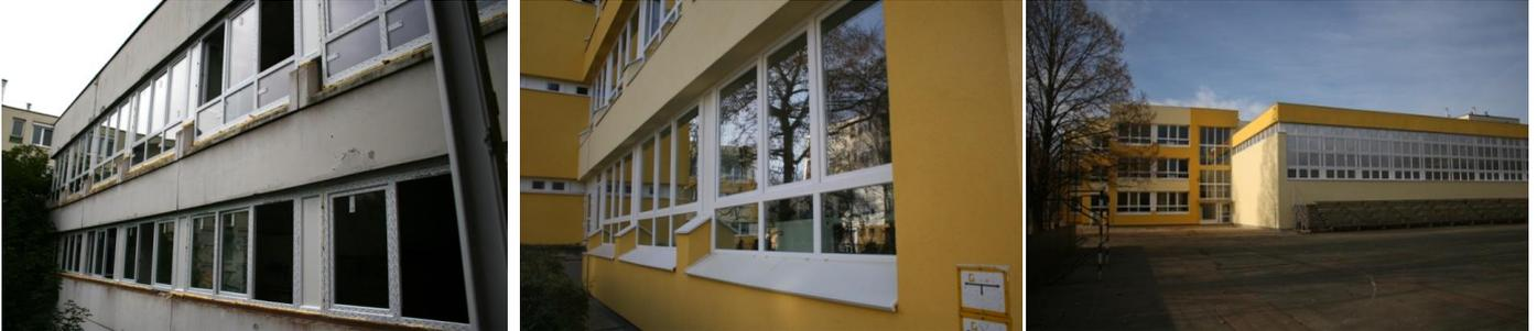
The structure of the buildings cooling surface and mechanical engineering structures do not meet current standards. The heat loss of the original doors and windows of the building were very high, the boundary heat transfer factors were higher than the current regulations.
